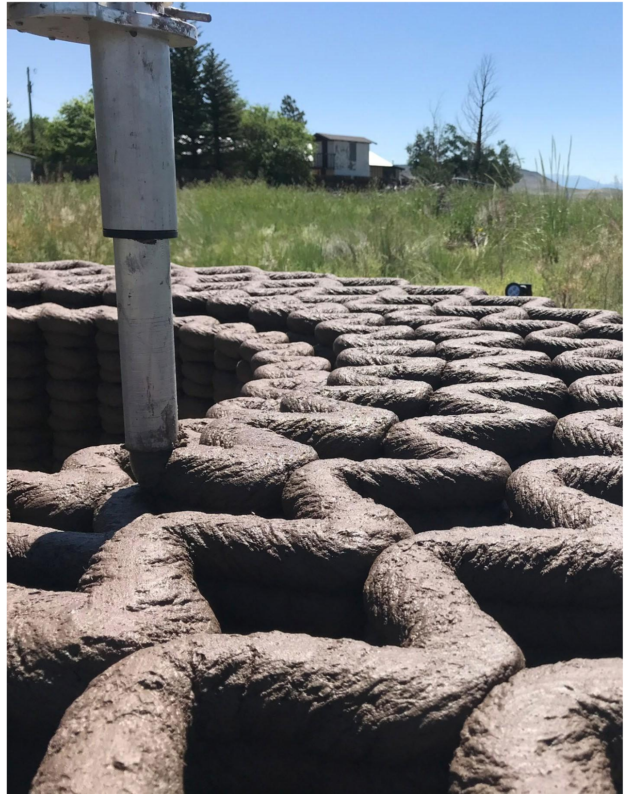
Mud Frontiers - Emerging Objects Raw earth structures printed with a portable robot
