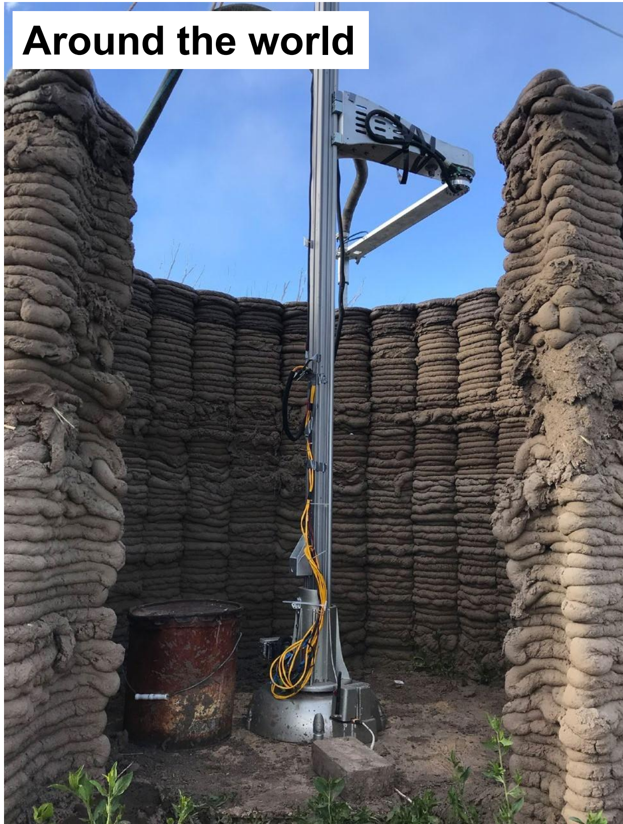
Mud Frontiers - Emerging Objects Raw earth structures printed with a portable robot
